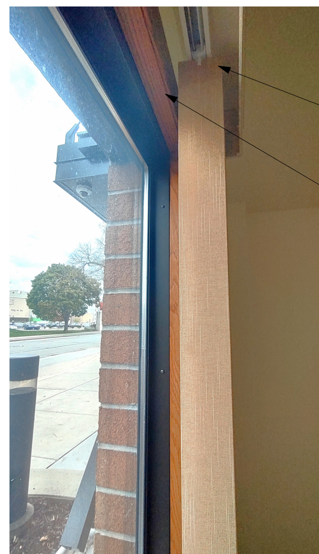
REMOVE EXISTING BLINDS AND HARDWARE REMOVE EXISTING WOOD TRIM
