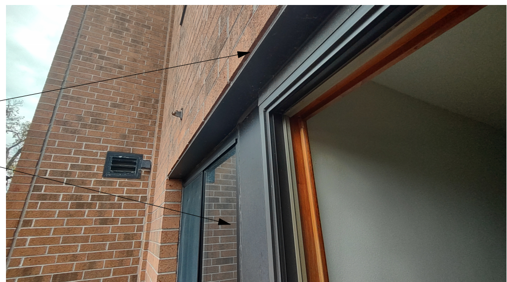
EXISTING LITTEL TO REMAIN GLAZING SYSTEM TO BE REMOVED
